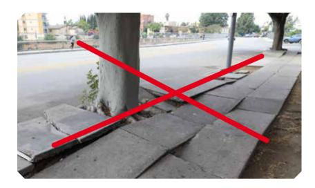
As trees grow, so does their volume of roots. As a result, the tree roots cause the soil to expand, which lifts the pavement. Even in structural soils, roots eventually push the stones apart too.
